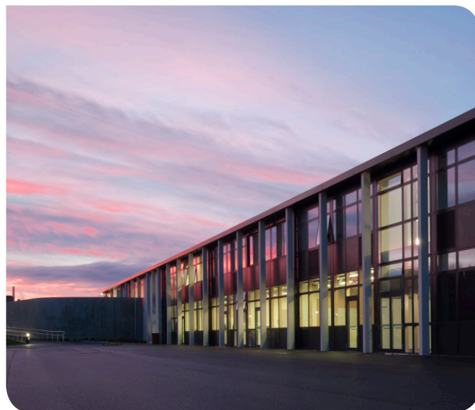
Photo courtesy of Donald MacLaren, Morrison Construction.
