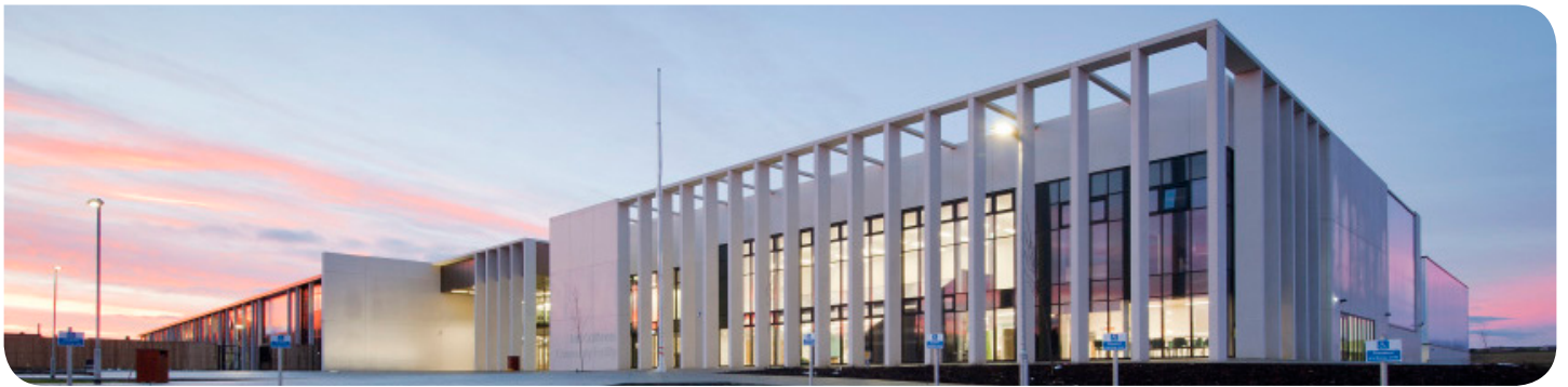
Photo courtesy of Donald MacLaren, Morrison Construction.
